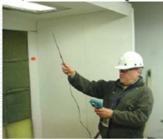
Airflow measurements indicate new spray paint booth exhaust system removes harmful paint
