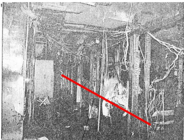
Fire develop by V shape in the basement floor.
